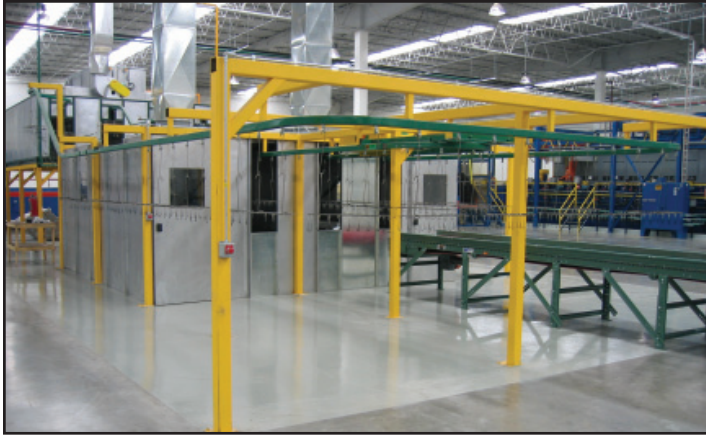
Dip/Drain line at the modern 50,000 sq. ft. plant in Warren, Michigan.
