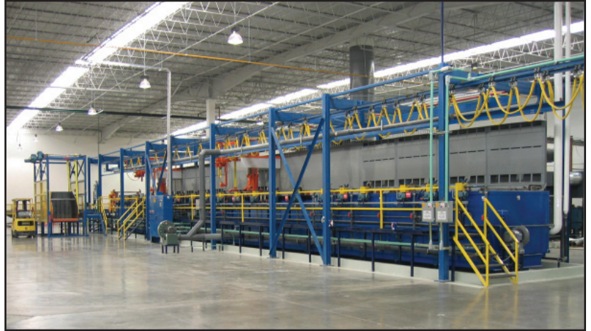
Hi speed zinc phosphate barrel coating line at the 66,000 sq. ft. plant in Queretaro, Mexico.
